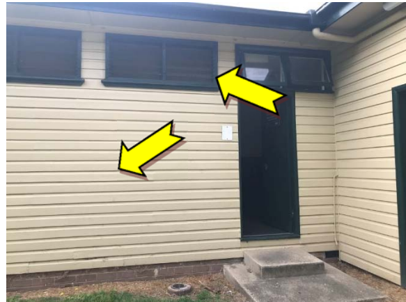
Photo 4. Exterior throughout, walls, window and door frames – suspected lead-containing yellow and green upper coloured paint systems.
