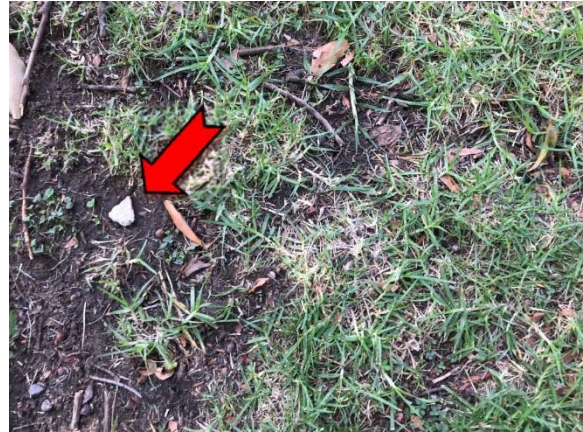
Photo 2. Exterior, throughout, ground – asbestos-containing fibre cement debris.
